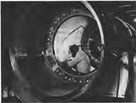
The airlock tunnel assembly was fabricated at the McDonnell Douglas facility in St. Louis. This photo shows the hatch still being tackwelded.
