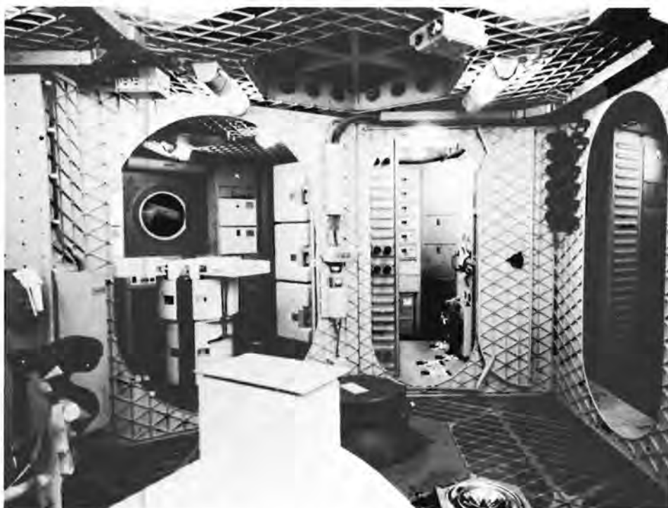
The overall interior of the crew quarters area in the Skylab High Fidelity mockup, at McDonnell Douglas, Huntington Beach, where the Workshop was fabricated. The sleep compartment is at the right, waste management compartment in the center, and the wardroom at left.
