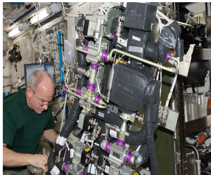
Crewmember performing maintenance on ISS CDRA
